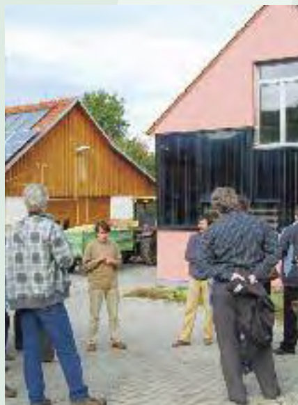
Centrum Veronica Hostětín: The first passive house of a municipality in the Czech Republic.
